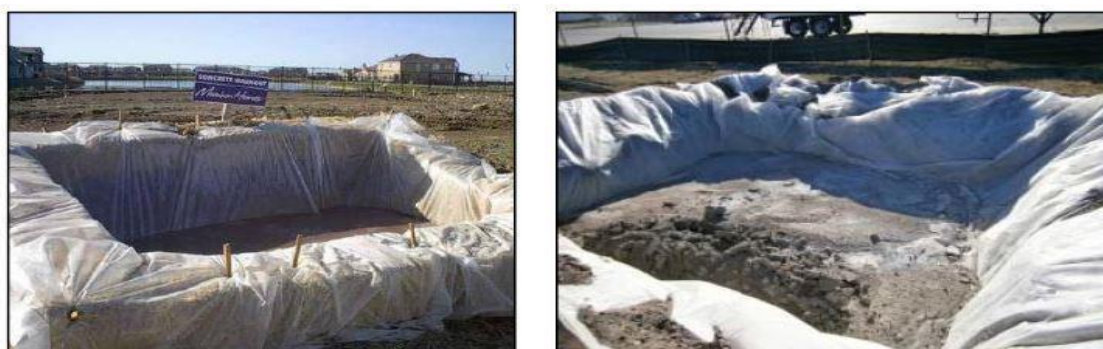
Figure 5.11.1- Example of a simple lined concrete washout skip
